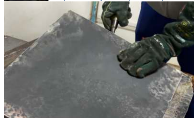
Figure 54 Remove the plastic tile carefully with a chisel or scraper
