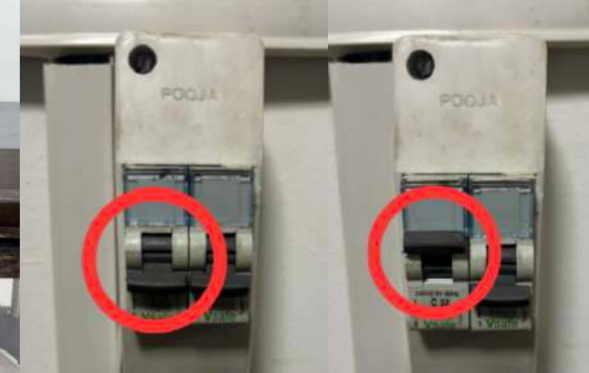
Figure 41 Switch in OFF position (left) and ON (right)
